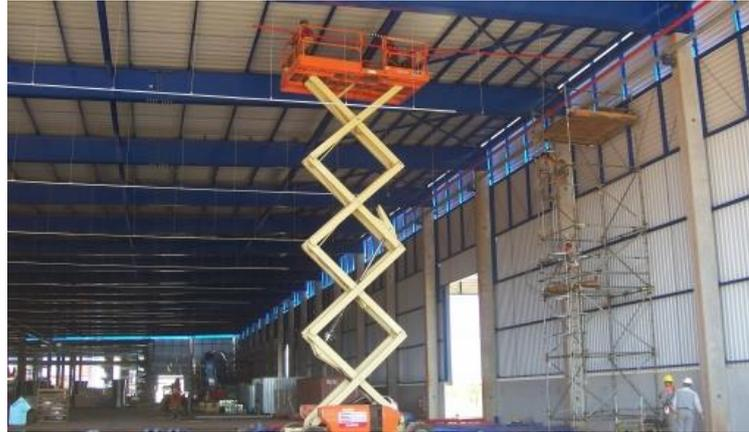
Figura 3 Plataforma Tesoura Diesel (MILLS, 2017)
